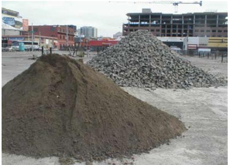
(Right) Piles of soil and rock used to make a structural soil mix for a project in San Francisco. The 6-inch cobbles proved too large to mix properly. 1-2 inch angular rock was substituted and the final mixture was installed. Structural soil using two-inch angular rock provides the best root anchoring due to better friction (personal communication with Claus Matteck).
